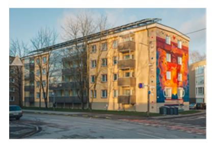
The **objective of the retrofitting** plan was to drastically reduce the energy usage of the demo area hrustsovkas. The average energy consumption of these buildings was before the retrofitting about **270 kWh per m2** annually and the target level is **90**, reducing energy consumption by more than **66%**.
